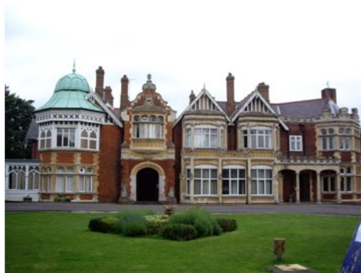
(a) Main building
